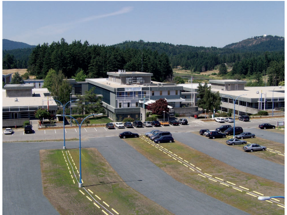
The 190,000 square foot facility at VITP.
