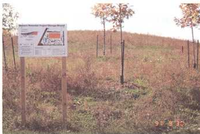
A close-up of the mound showing the sign and environmental monitoring chart.
