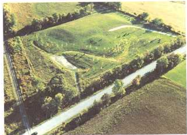
Passmore Avenue Site after construction of interim storage mound. (1997)
