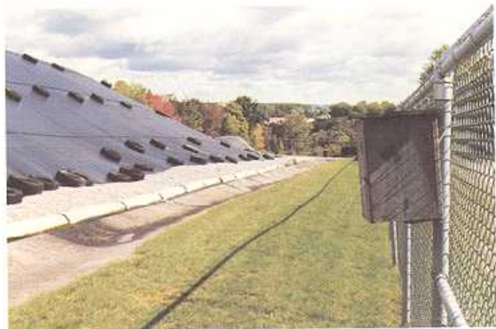
Environmental monitoring station at historic waste storage site in Port Hope.
