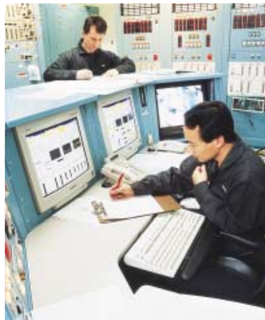
Inside the control room for the MAPLE Unit 1 reactor.
