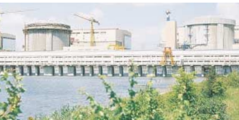
AECL is negotiating to complete Unit 2 at the Cernavoda site in Romania.
