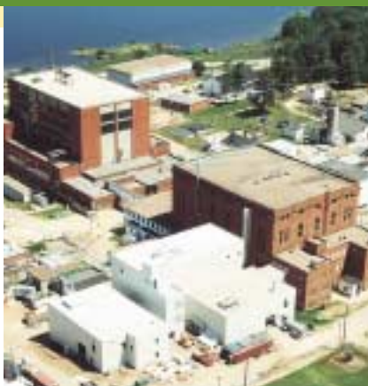
Seen in the foreground, an exterior view of the buildings housing the two new MAPLE isotope production reactors and associated processing facility at Chalk River.
