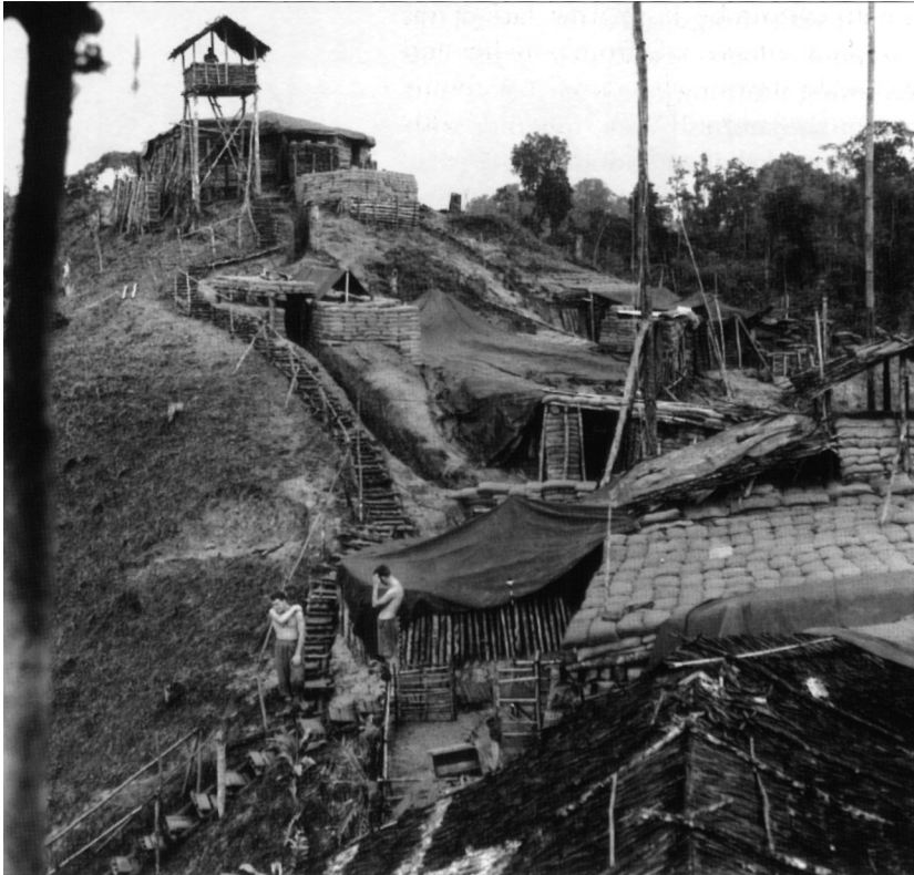
A typical border fort in Sarawak. It has an observation tower, bunkers made of logs and sandbags linked by communication trenches, and a stepped walkway up the hill—essential in the muddy conditions created by tropical rainfall—made of cannibalized ammunition boxes. Note the tall poles supporting radio aerials, and the vegetation cleared away to provide good fields of fire.
