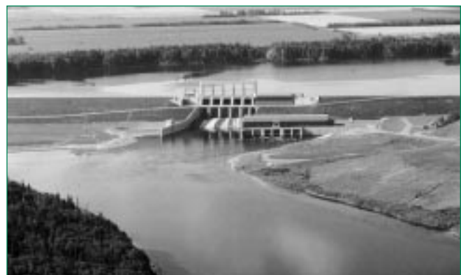
Hydroelectric Generating Station
