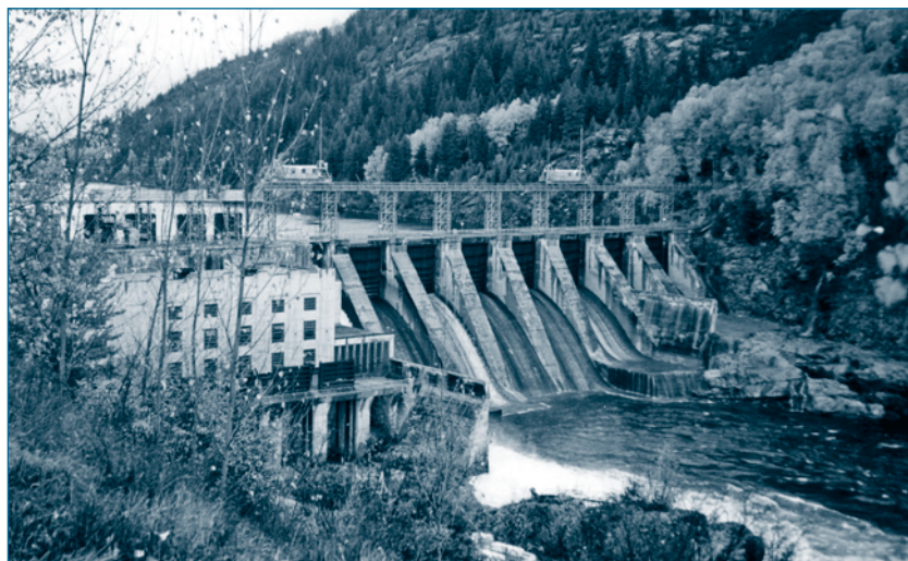
Columbia Power Corporation's Brilliant Dam on the Kootenay River, near Castlegar, B.C.
