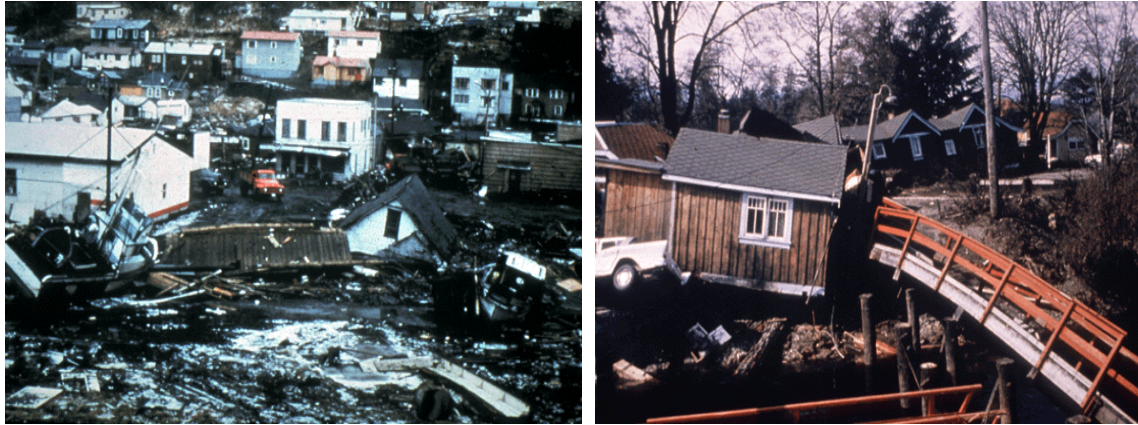
Figure 6 Tsunami effects in Port Alberni, 28 March 1964 (Source: British Columbia, 2003a)
