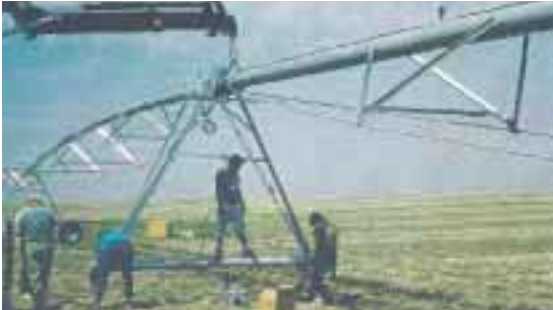
Economic development gathers steam in the Alberta Region. Irrigation Pivot under construction at Siksika Nation.
