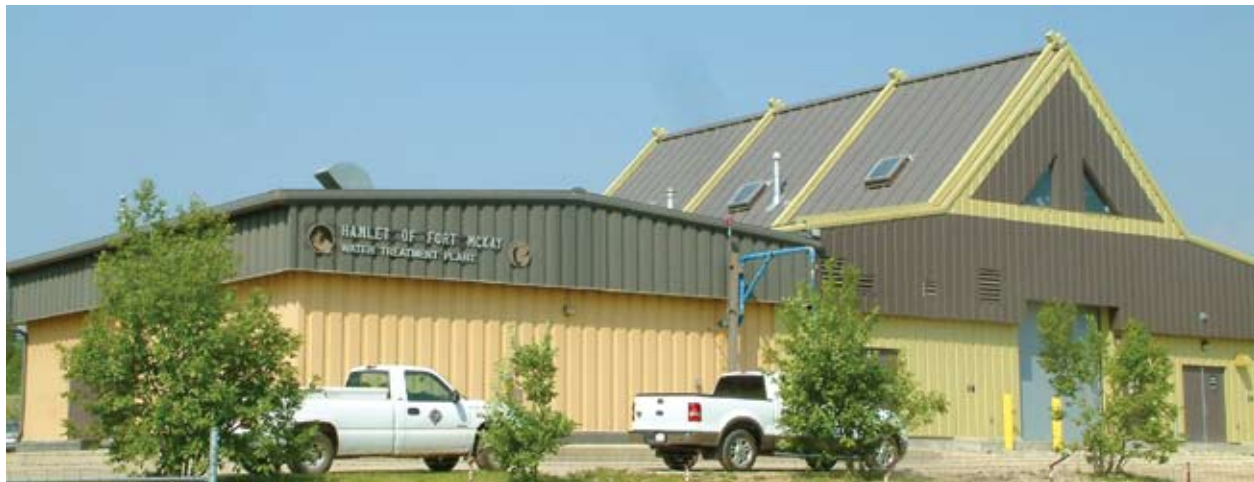
ABOVE: Fort McKay water treatment plant
