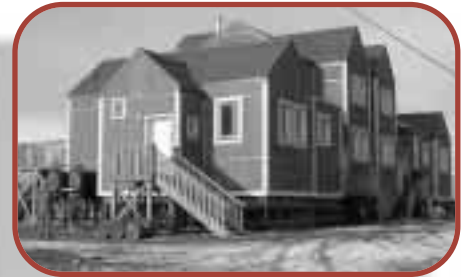
New housing going up in Arviat.
