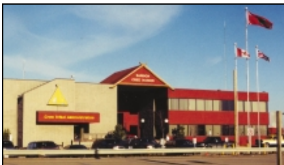
Samson Cree Nation Administration Building
