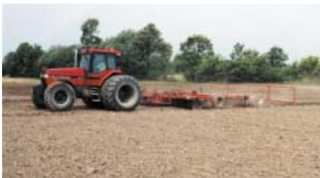
Large project sites can be prepared with standard farm equipment such as this combination of plow, disc and harrow. Kim Delaney
