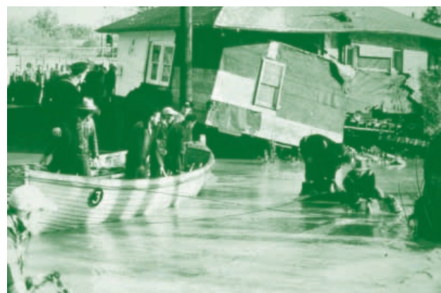
Hurricane Hazel – flood damage and rescue
