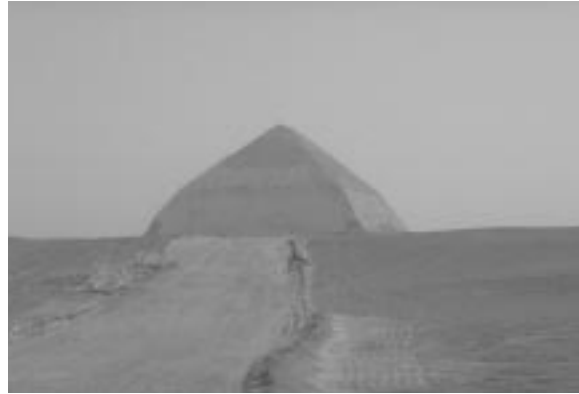
The Bent Pyramid was built by the pharaoh Snefru. During construction, the engineers realized that the top half had to be bent inward to prevent the whole structure from collapsing. CMC S97 10630
