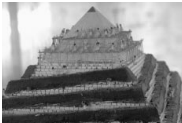
Ramps were used to haul stone blocks on wooden sleds up the sides of the pyramids
