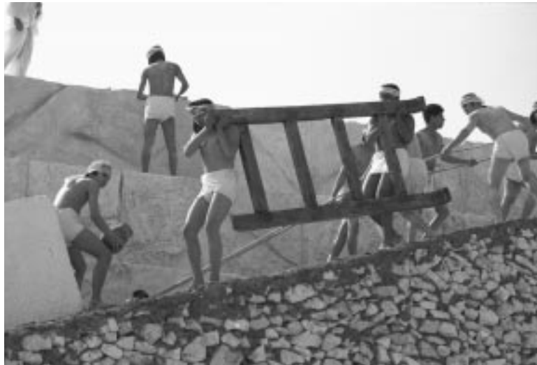
Water was sprinkled under the sleds to lubricate the ramps, making it easier to move the heavy stone blocks. Re-enactment scene from the film Mysteries of Egypt.
