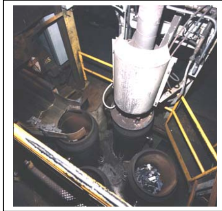
Scrap preheater showing scrap loading position (far left); preheating station (top); and scrap bucket pick-up station (right)
