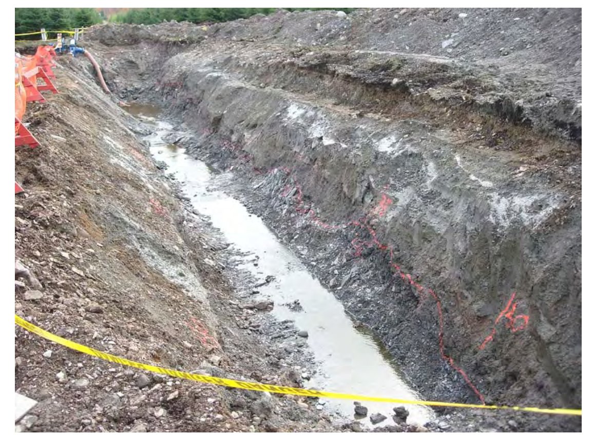
VIEW OF TRIAL EXCAVATION TR-B-05 LOOKING SOUTH
