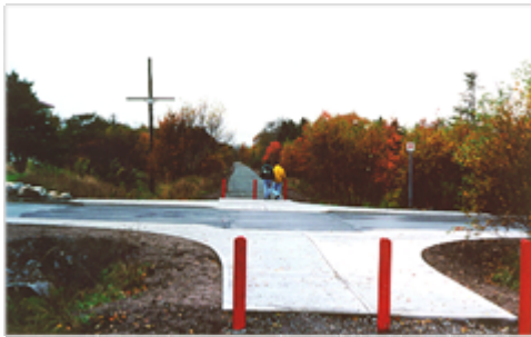
“Before” and “after” photos of an at-grade intersection of the Newfoundland T’Railway and a local road
