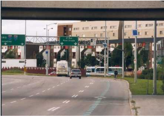
Reserved bus lane, De La Couronne Street.
