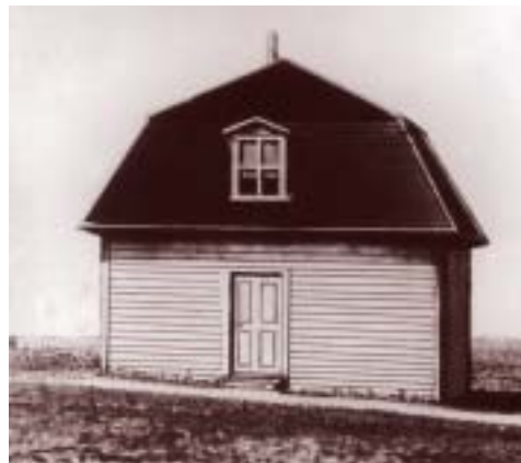
The first hospital in Western Canada, built by the Grey Nuns in 1871
