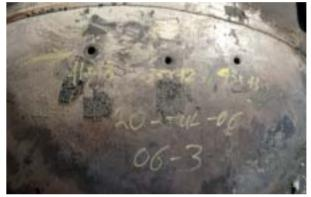
Figure 10 – Drain Holes in End of Tank 06-3
