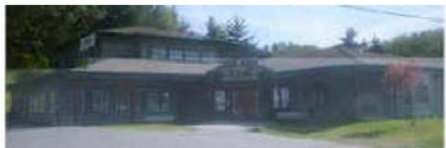
Tsawout First Nation Administration Office
