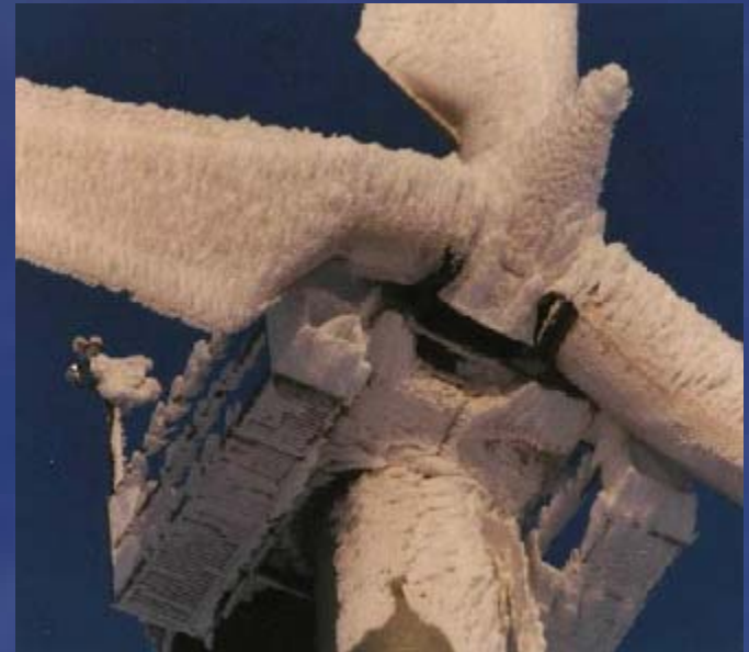
Bonus Heated Bearing Anemometer (30 m) (replaced in first year)
