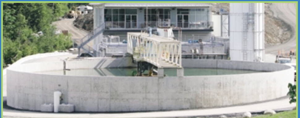
Britannia Mine Water Treatment Plant
