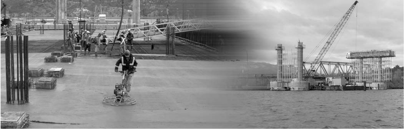
William R. Bennett Bridge Project
