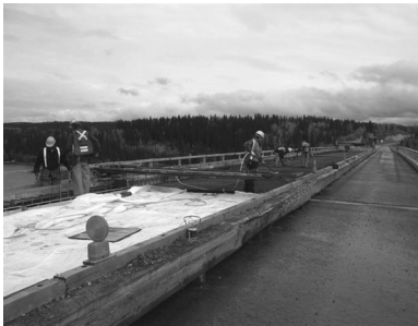
Workers replace the Teslin River bridge deck.
