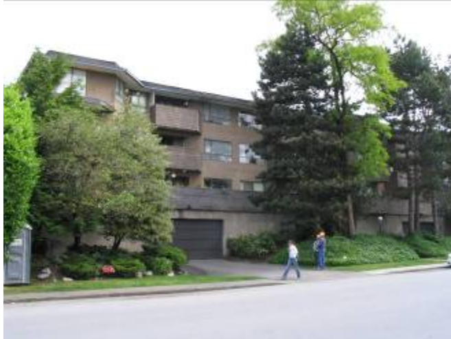
Figure 1: South side (front) of building.
