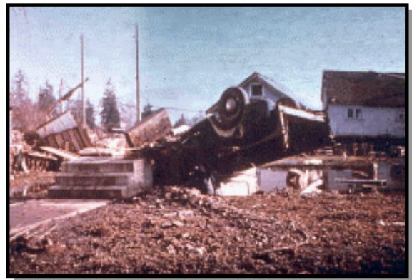
Damage caused by tsunami in Port Alberni, 1964. The power of a tsunami is exemplified as automobile replaces home in this central Vancouver Island community. — Provincial Emergency Program, Government of BC
