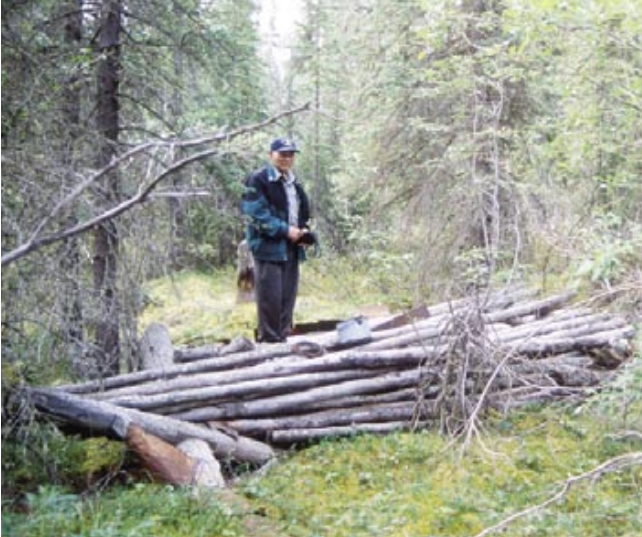
Collapsed log cabin-style cache.
