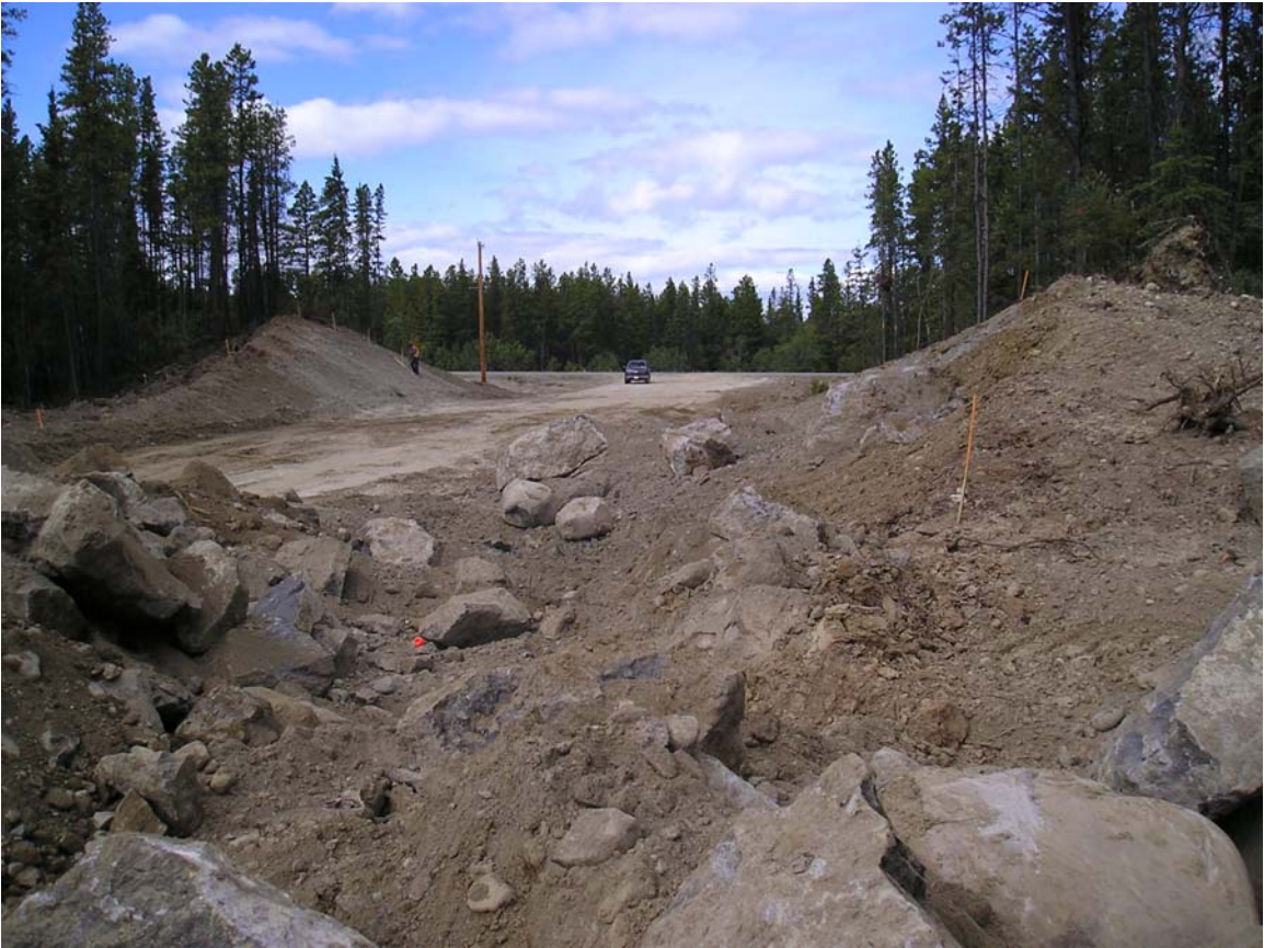
Rock Outcrop #1 on Levich Drive Adjacent to Lot 18 After Blasting – August 2006
