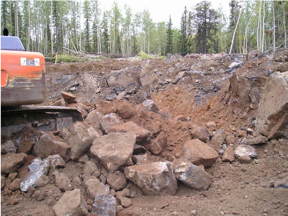
Rock Outcrop #3 on Collins Lane Adjacent to Lot 40 After Blasting – August 2006
