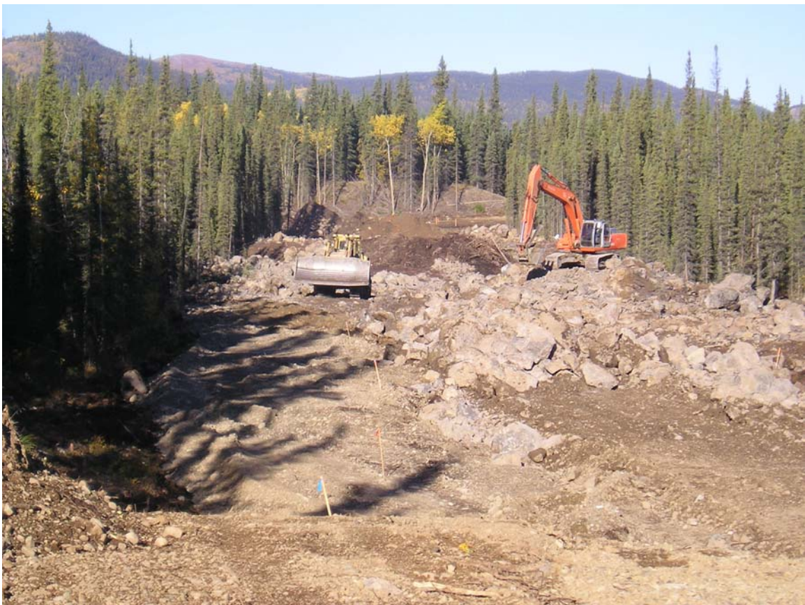
Rock Outcrop #4 on Talus Adjacent to Lot 24 After Blasting – August 2006
