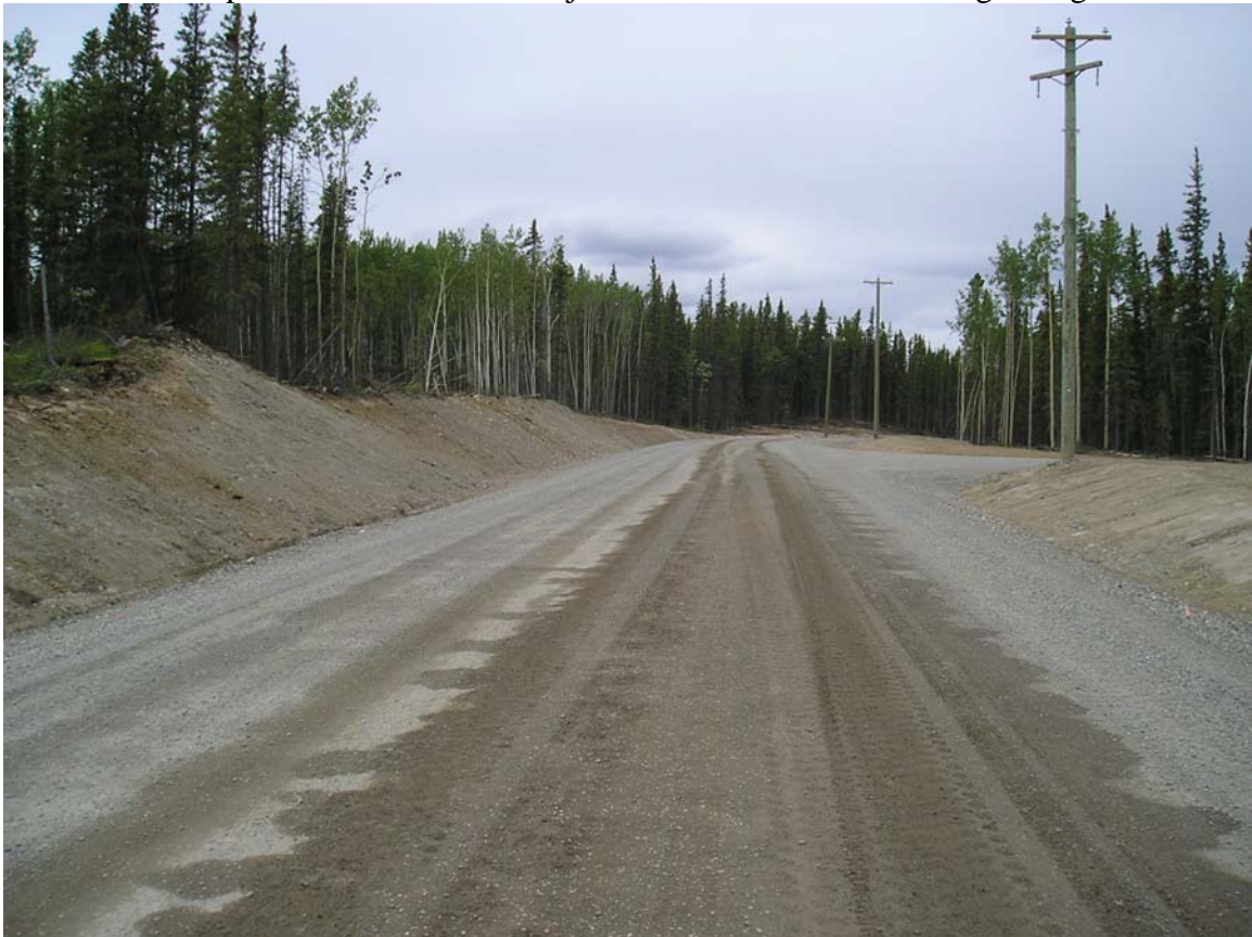
Rock Outcrop #3 on Collins Lane Adjacent to Lot 40 After Clean Up - July 2007
