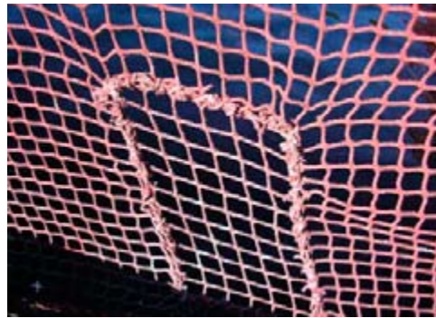
Net repair completed on the jump net portion of a containment net.
