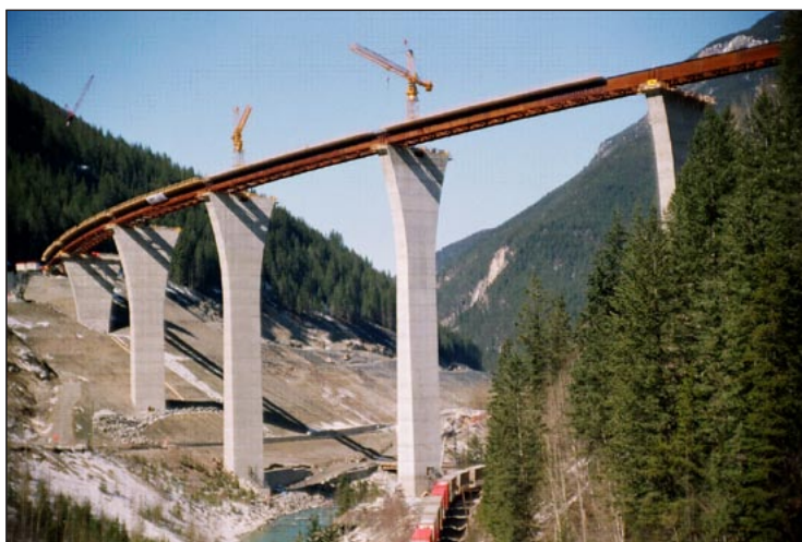
Park Bridge construction
