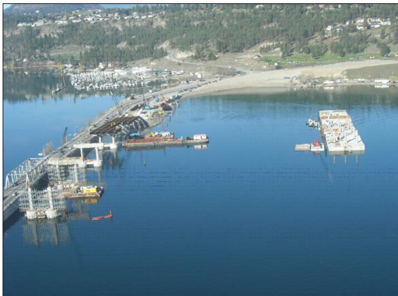
Bridge site construction
