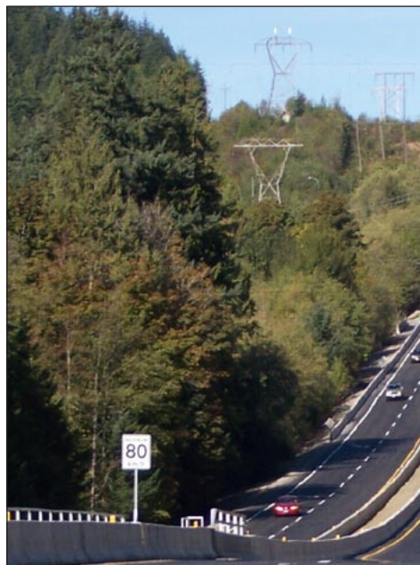
Completed section at Furry Creek
