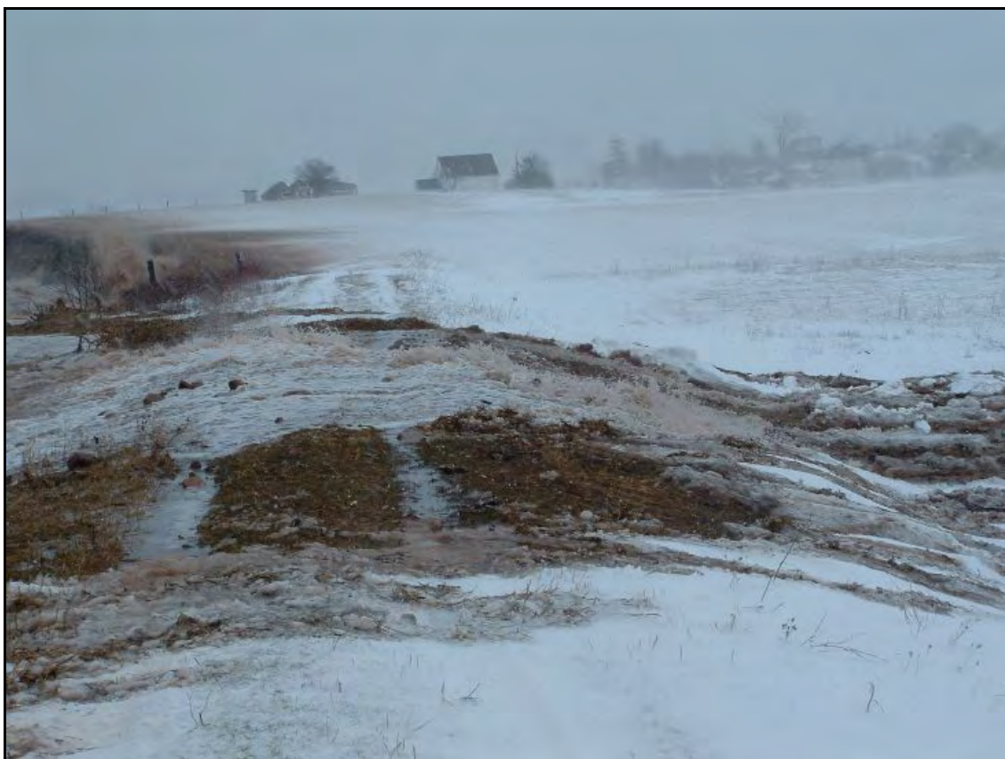
Figure 2.6: Storm impacts on Feb 1, 2006 at the Avonport Dyke. a) storm waves battering marsh; b) storm surge reached upper limits of dyke and dyke overtopped. Photo by T. Hamilton, 2006.
