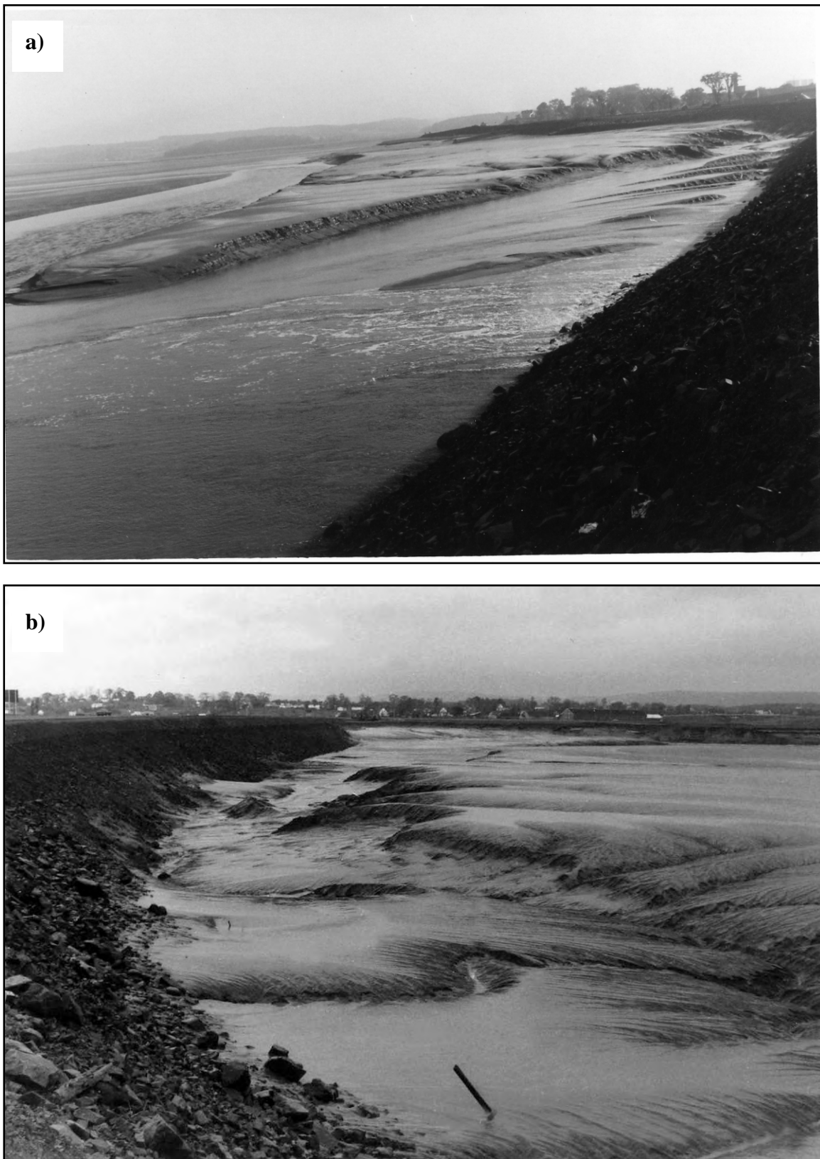
Figure 2.23: Rapid accumulation of unconsolidated sediment close to the causeway. a) Development of what appears to be a mud point bar in Oct 1970 near eastern end of causeway, 3 months after the construction was completed and b) infilling of channel parallel to the causeway in Nov 1970. The future 'causeway' channel is likely the one visible in photo 'a' top left (photos from MMRA, 1970).
