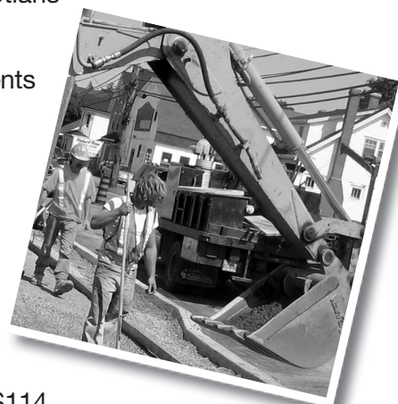
Sanitary Sewer Replacement Bible Hill-Municipal Rural Infrastructure Program
