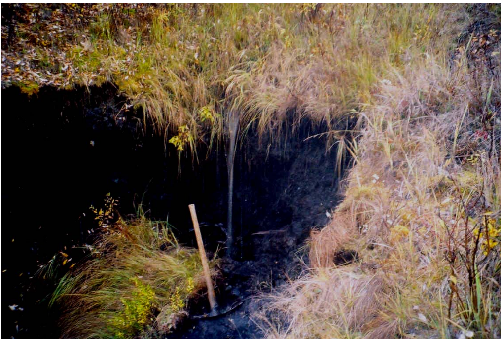
Top of cut prior to any construction, flow estimated at 3 to 4 litres/second, Sept 6 th , 2006
