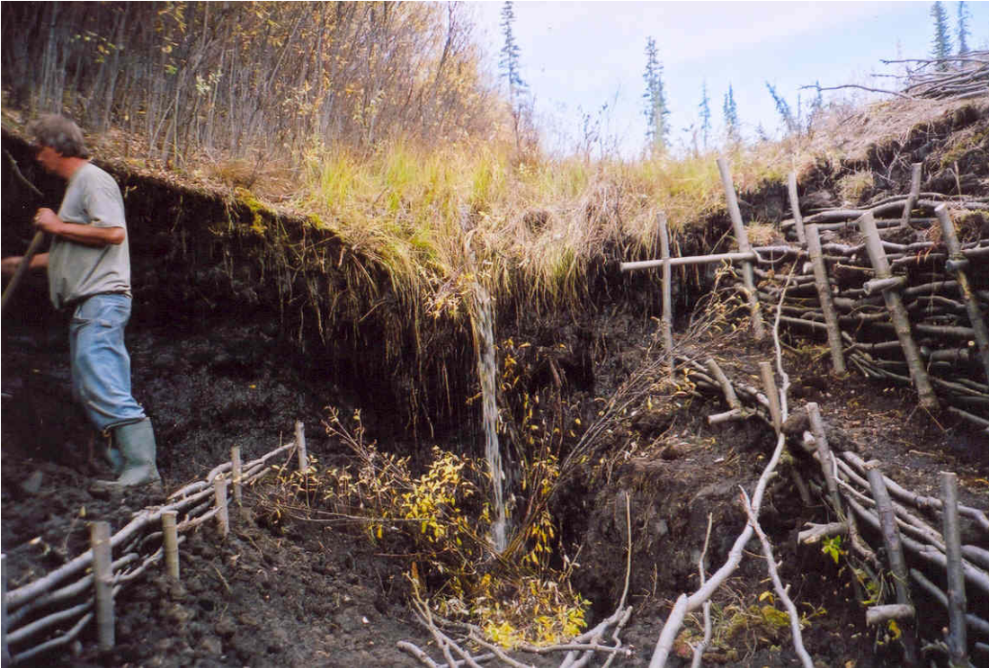
West wall construction, September 7 th , 2005.
