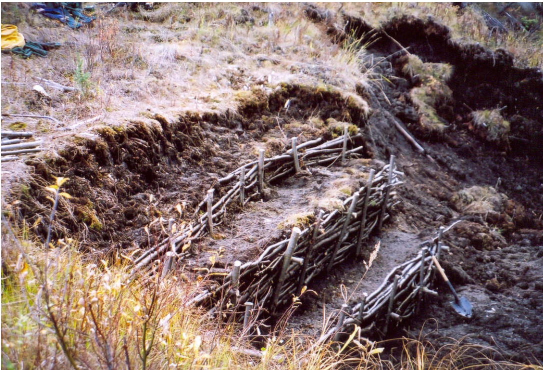
East wall completed, looking down the cut. September 7 th , 2005.
