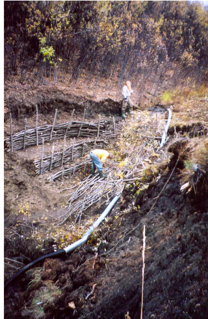
Completed live willow flume and retaining walls, with both September 9 th , 2005.
