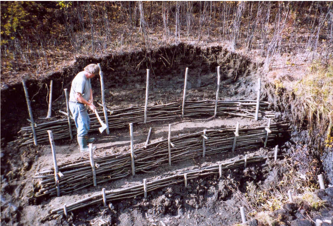
Working on final tier on the west wall, September 8 th , 2005.
