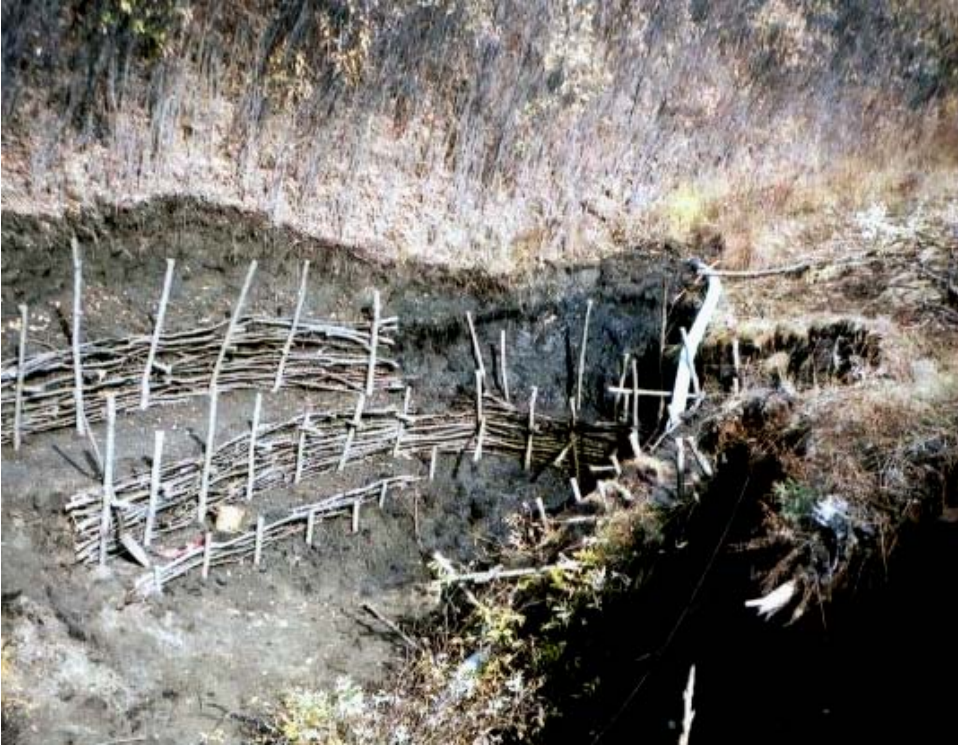
First retaining wattle fence completed on rear wall, September 9 th , 2005.
