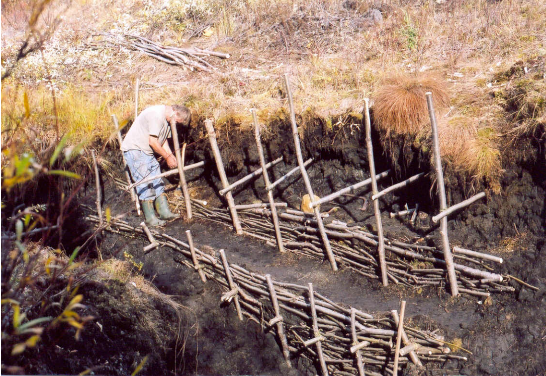
Constructing second tier on the east wall. September 6 th , 2005.
