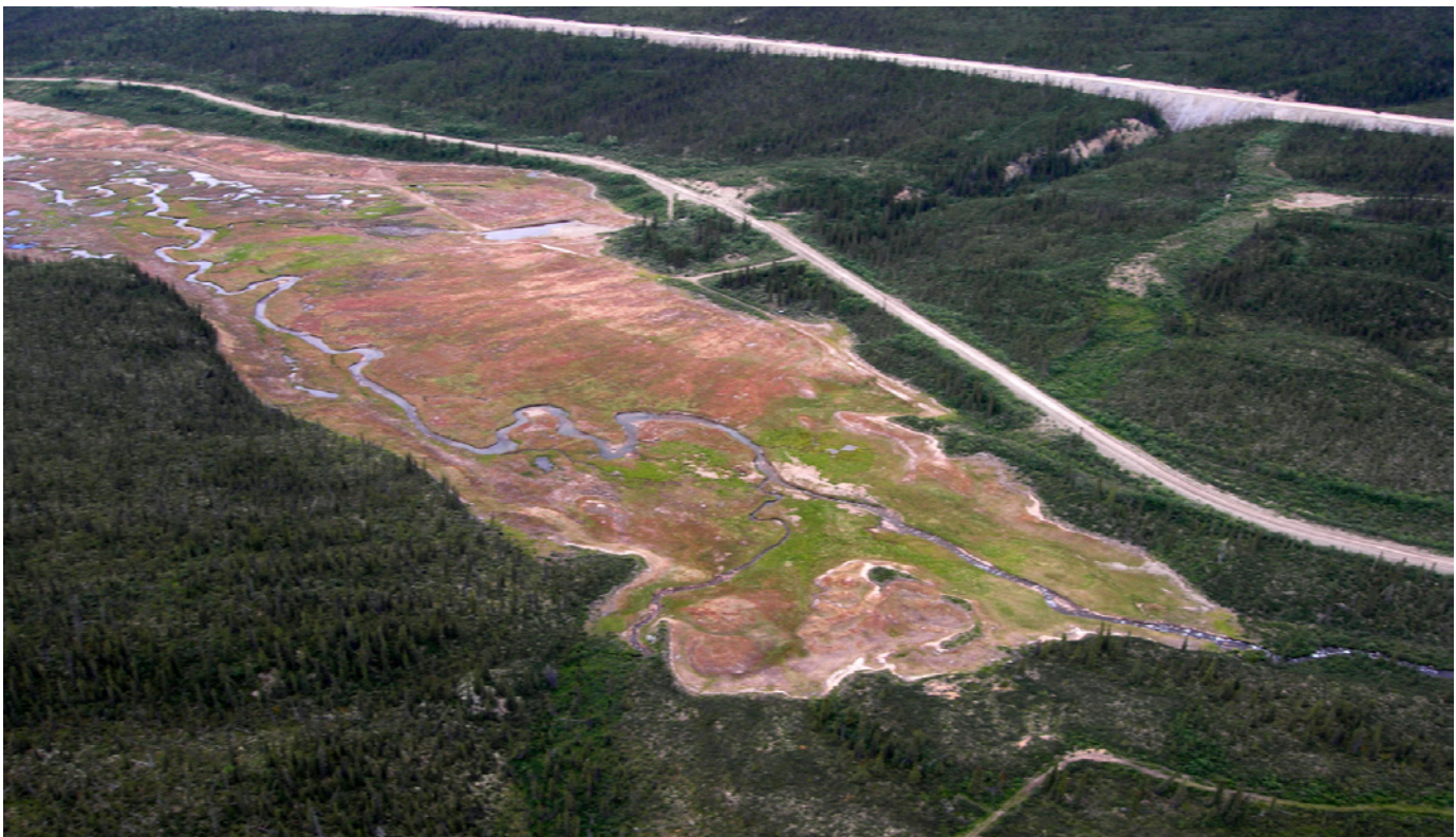
Figure 3. Reclamation of fresh water reservoir and supply dam, Faro, Yukon.
