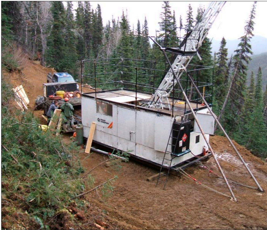
Figure 37. Drilling at the Tootsee River tungsten-molybdenum project.
