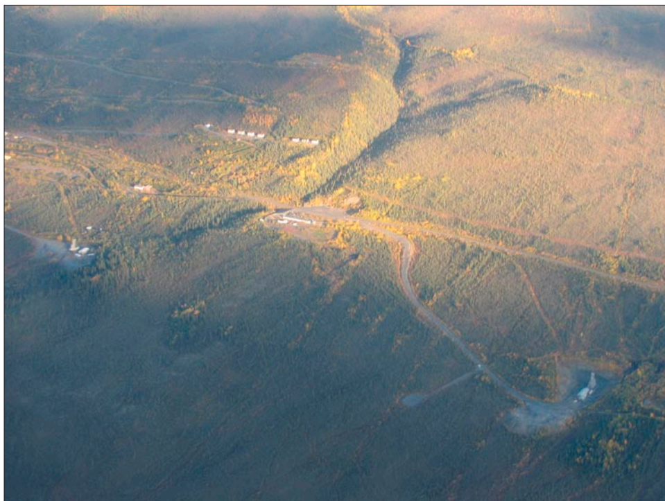
Figure 23. View of the new exploration camp (centre) and the headframes of the Husky mine at the western end of the Keno Hill silver camp.
