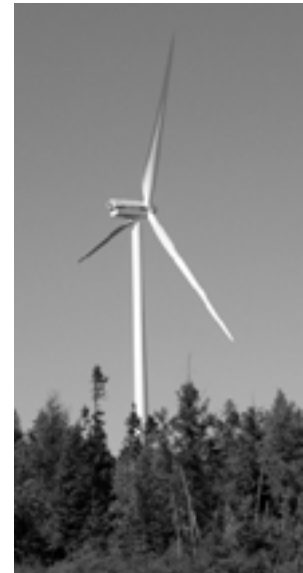
The largest wind turbine in North America, the V-90 produces about one per cent of PEI's electricity.
