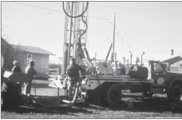
Figure 7. Test drilling to locate groundwater aquifers
