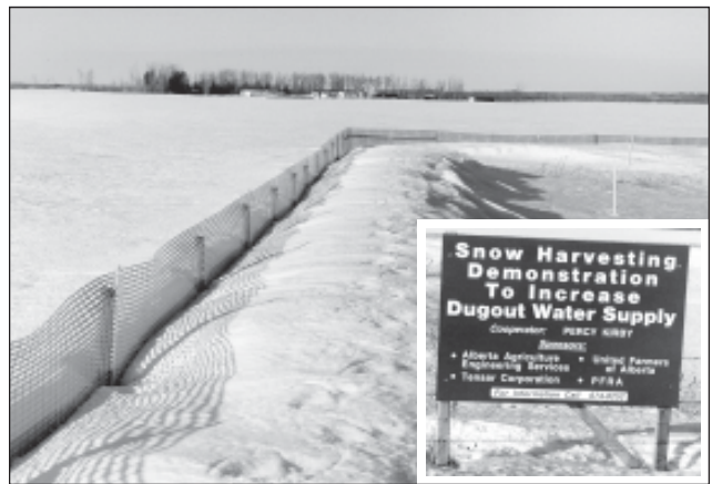
Figure 4. Plastic snow fence placed around the perimeter of a dugout
