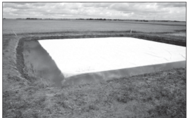
Figure 5. Plastic cover to reduce dugout evaporation losses
