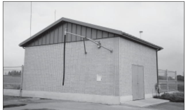
Figure 6. Tank loading facilities
