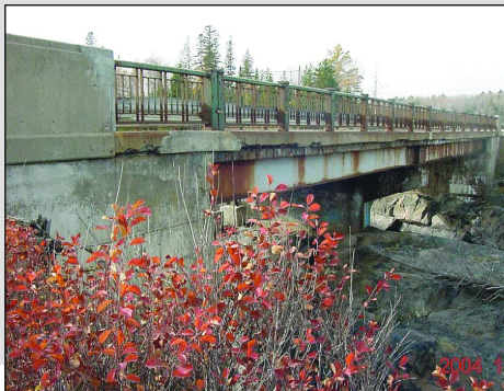
Highway 144 project "before"
