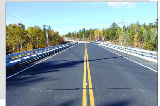
Highway 11 project "after"
