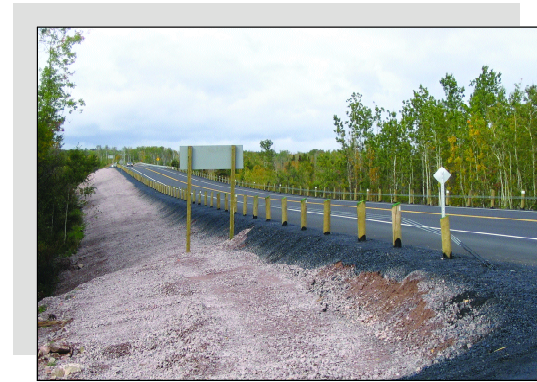
Highway 11/17 project "after"
