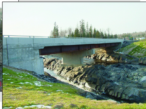
Highway 144 project "after"
