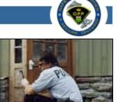
All exterior doors should have escutcheon plates with back plates or wrap-around door channels installed around any deadbolt lock. Plates are to be secured from the inside with 1.9 cm (3/4 inch) carriage or hex bolts that cannot be removed from the exterior. The small screws that are supplied with most escutcheon plates should be replaced with bolts. the holes in the (Redrilling escutcheon plate may be required.)
