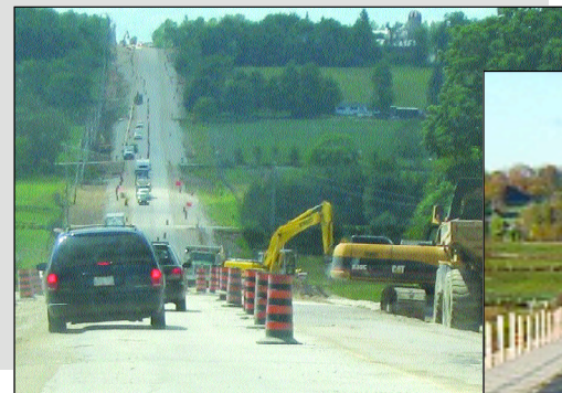
Highway 26 project "during"
