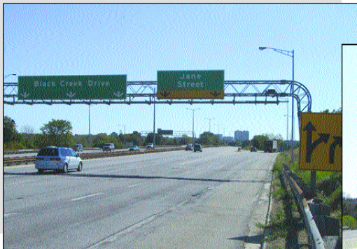
Highway 400 project "before"
