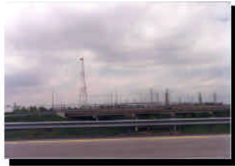
A' - VIEW TOWARDS HYDRO SUBSTATION
