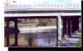
SITE 4, RIDEAU CANAL LOOKING SOUTH
