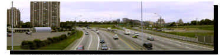
17 - LEES AVENUE OVERPASS CORRIDOR WEST
