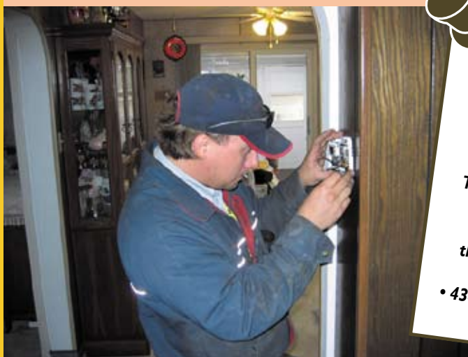
A SaskEnergy Network Member in Swift Current installs a programmable thermostat.
