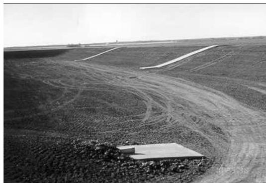
Earthen manure storage facility under construction
