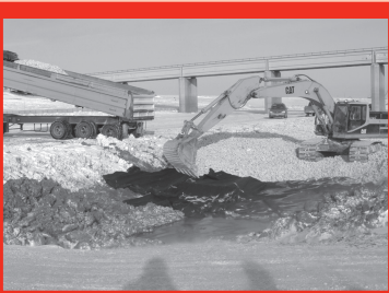
Erosion protection measures for the low flow channel
