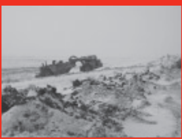
Excavation of Floodway channel
