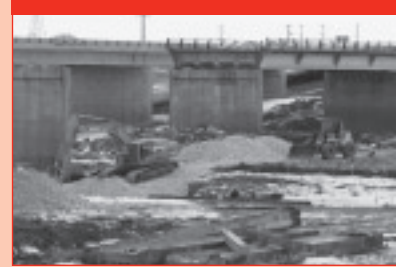
Demolition of southbound crossing of PTH 59 south bridge nears completion.
