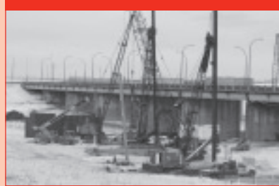
Driving piles at the Trans-Canada Highway #1 bridge site
