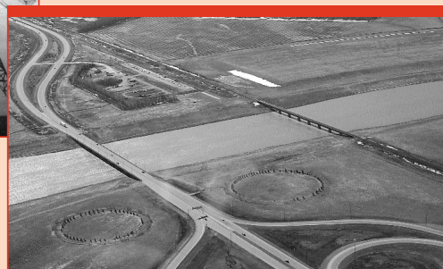
Rail & highway bridge upgrades
