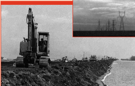
Construction of the West Dike
