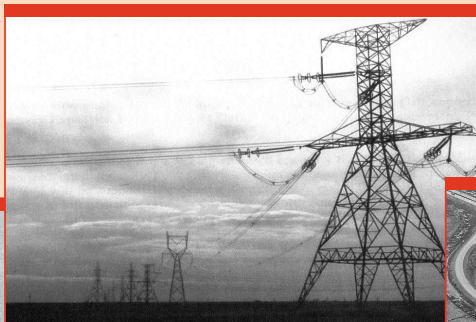
Modifications to transmission lines
