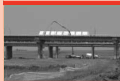
Cement pour for the bridge deck on the PTH 59 South Structure.
