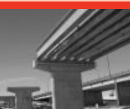
Installation of bridge girders on the new Trans-Canada Highway Bridge East.
