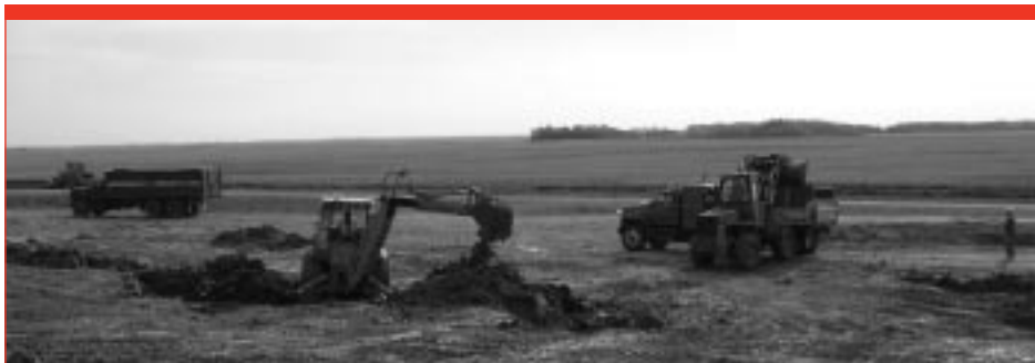
Access to earth depot located beside the St. Mary's Road Bridge.
