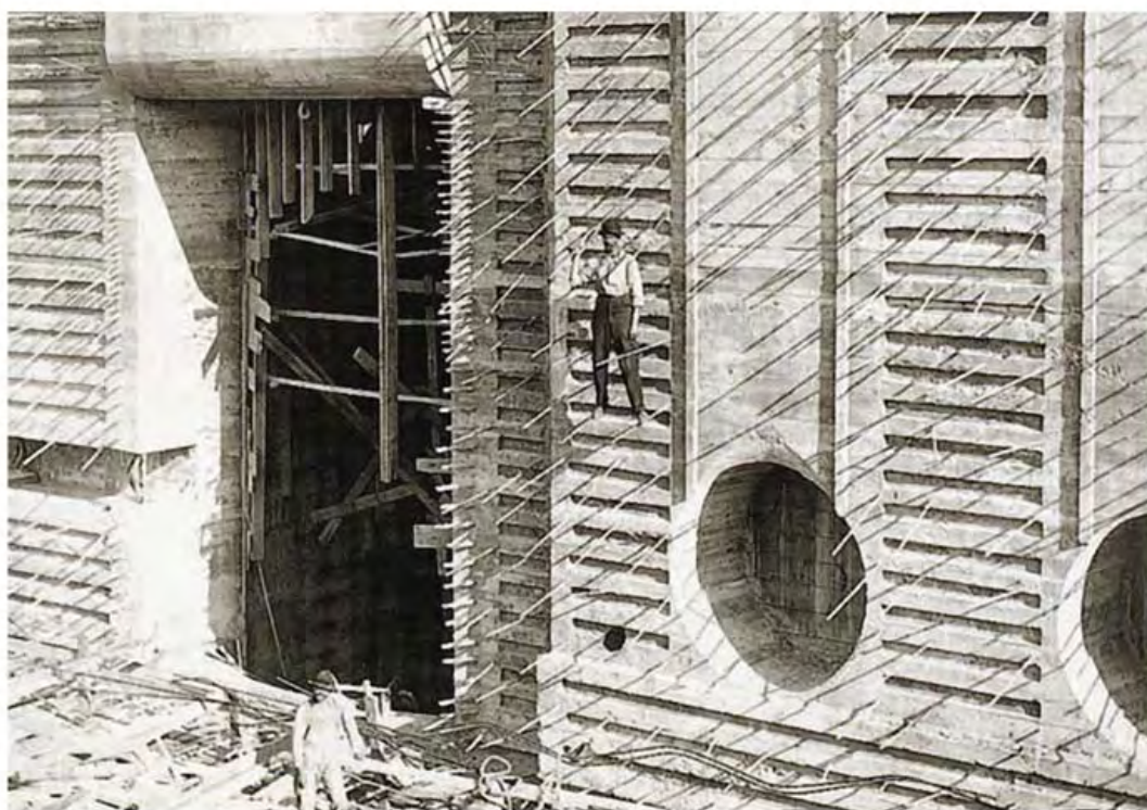
Construction at Pointe du Bois
