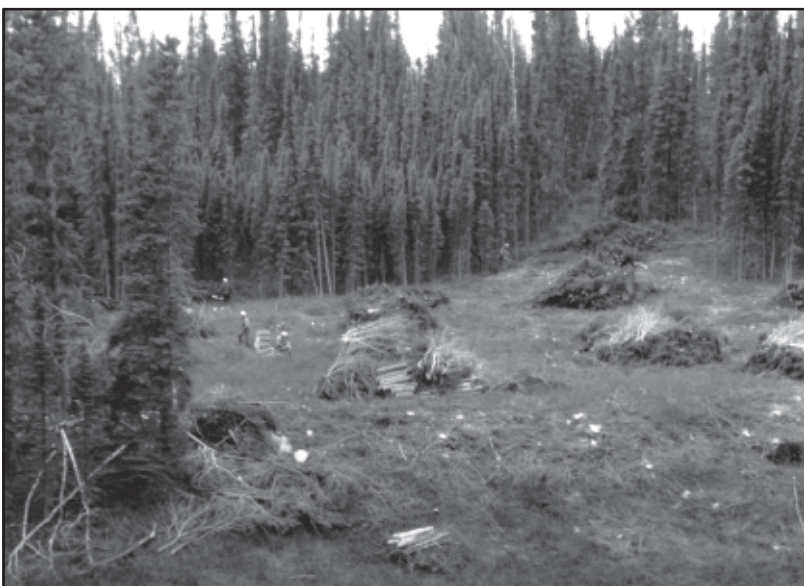
Slash is piled and burned during construction to avoid future forest fire hazards.
