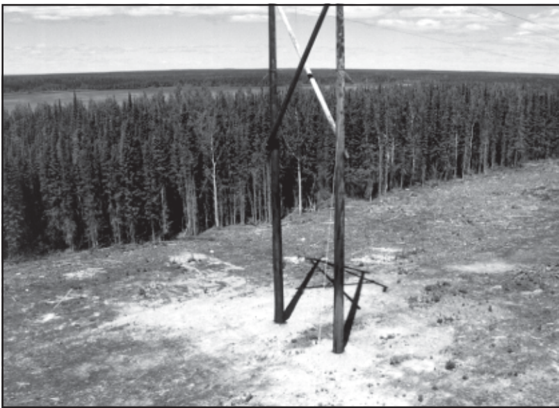
Gulfport structure on a stable non-eroding terrain type.
