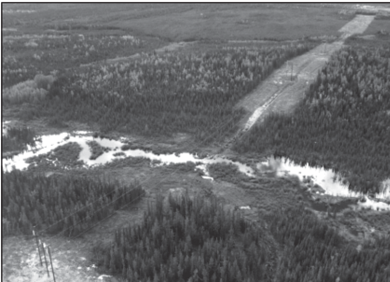
Buffer zone left on a right-of-way to protect a river valley.
