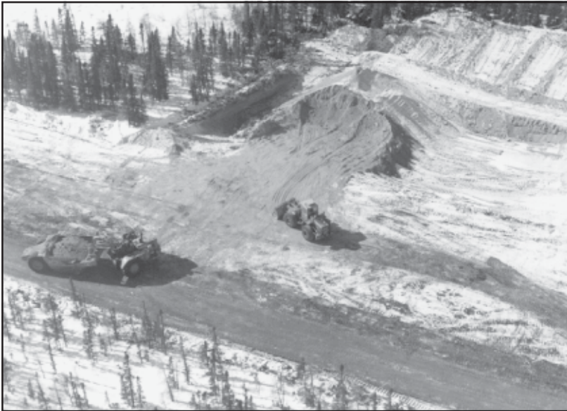
Borrow pit for construction
