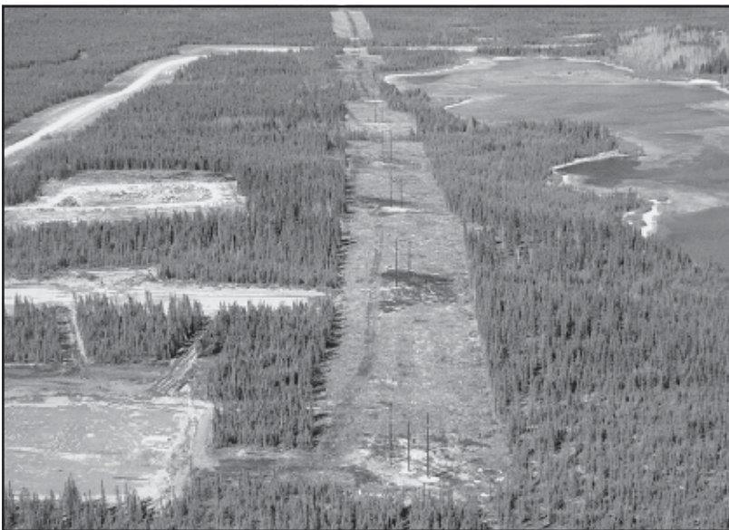
Transmission line in Northern Boreal Forest
