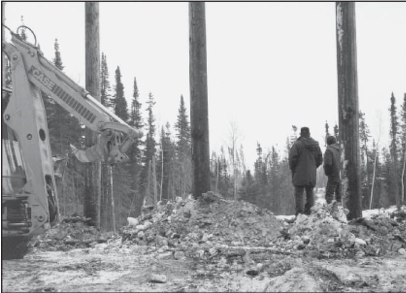
Construction noise is short term.
