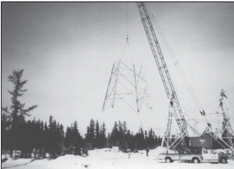
Construction site in northern Boreal Forest
