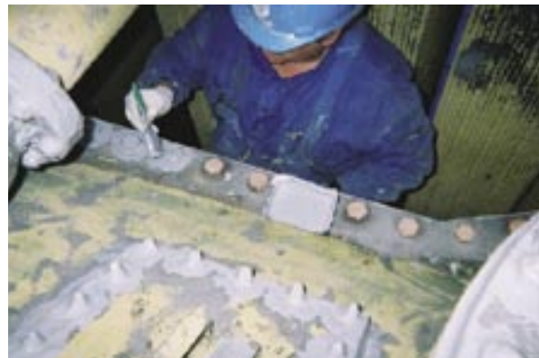
Applying encapsulation sealant to joint surfaces on a transformer
